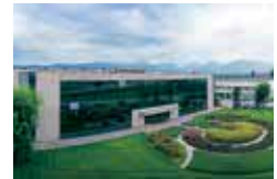
The New Factory
