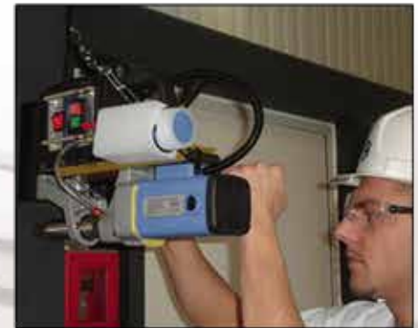
Kernbohren in allen Lagen Core drilling in all positions
